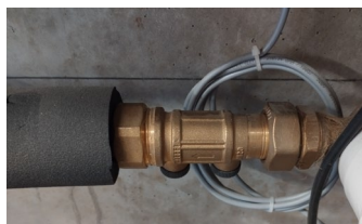
Figure 27 Clapets anti-pollution de type EA
