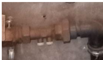
Figure 27 Clapets anti-pollution de type EA
