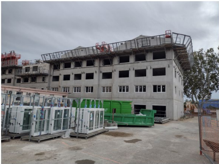
Avancement 80% cloisons PF
