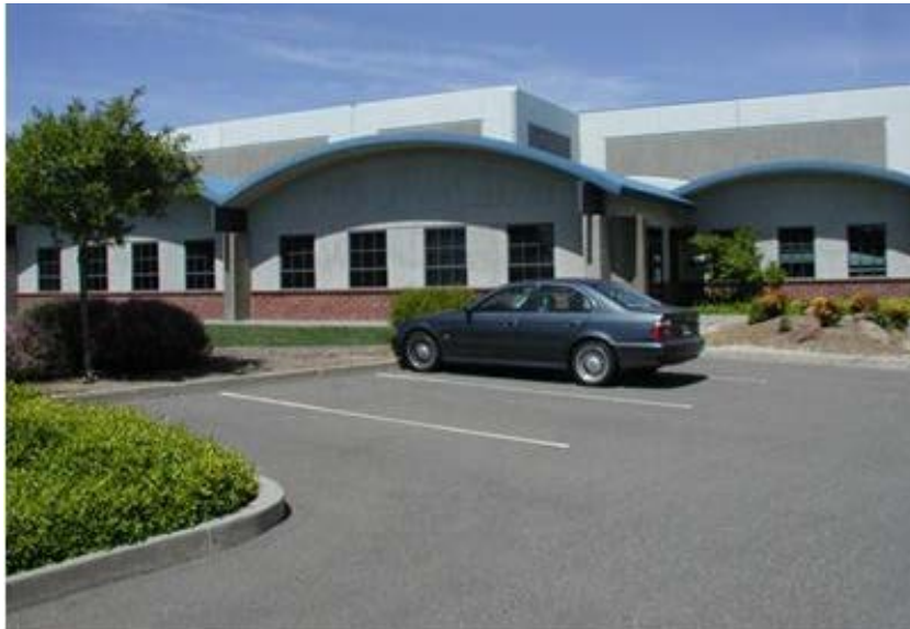
Tilt-up with barrel-roof offices
