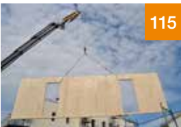
Transformation through a production system
